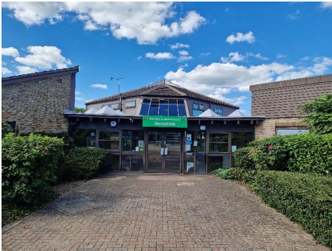
This is the main reception area.
